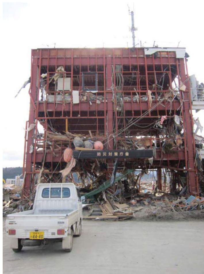
Disaster management center in Minami Sanriku
